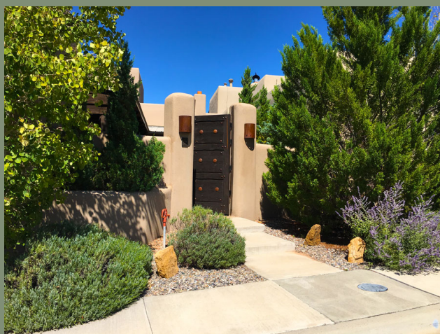
Courtyard home in Aldea .
